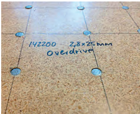
ABOVE: Ring shank nails securing 4.8mm hardboard type HB.H oil-tempered
