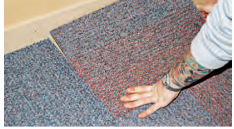
ABOVE: Take care with bitumen-backed tiles not to mark the skirting.
