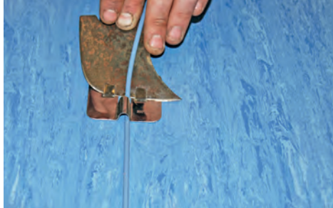
ABOVE: Trim the weld with so that the weld cools more quickly
