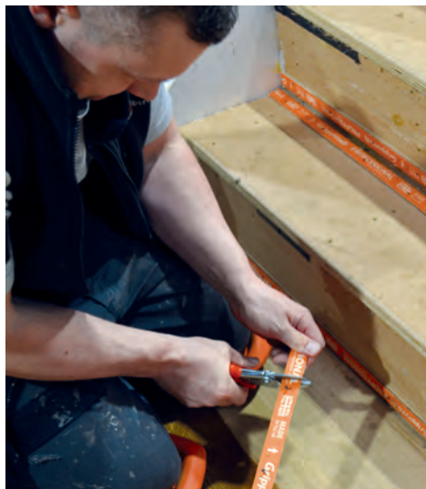
ABOVE: On stairs, the gripper should be the full width of the stairs and placed twice the thickness of the carpet away from the tread and riser where the tread and riser meet, if the carpet is being fitted as a continuous run.
