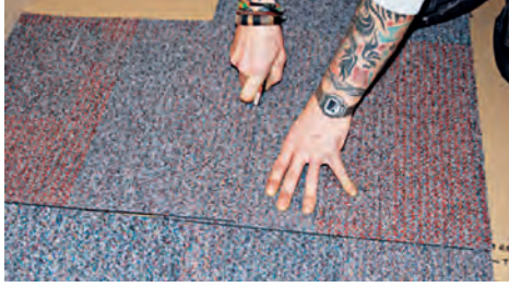
ABOVE: Fitting the tile using the back-cutting method
