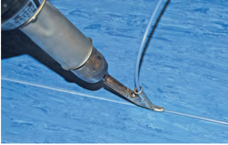
ABOVE: Apply the weld with a welding gun set at the correct temperature
