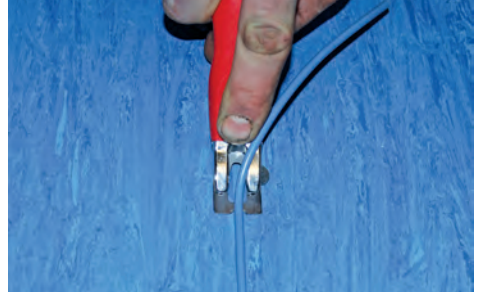
ABOVE: Mozart trimming knives makes trimming the weld easier and the changeable blade means no sharpening
